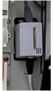
Temperature and humidity sensor
